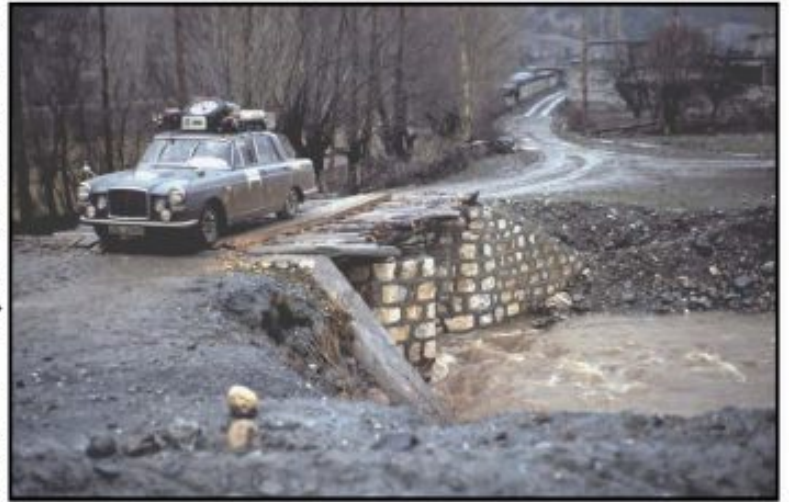
Bridge under construction!
